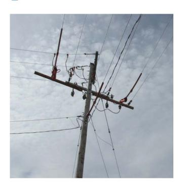
This also could be as complex as phasing in a three phase side break and jumpering onto the new and then removing jumpers from the old.
