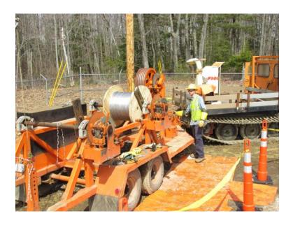
Concerning a trailer with only brakes on the reel, pulling wire smoothly is harder to achieve as the wire size gets larger. The trailers with Schematics (Bull Wheels) and multiple brakes can help with this problem.
