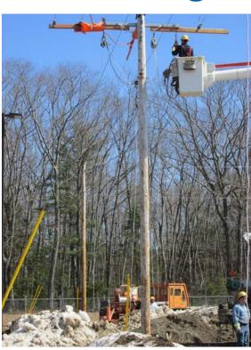
The first step is to get the wire in the shoe on the Wire Trailer end and rigged to the middle of the pole if necessary as to not twist the new arm. Then slack can be let into the wire by releasing the brakes on the Wire Trailer and the conductor can be cut to the ground. Then the Rope Trailer can be called and with the wire still hooked to the rope trailer pay in and get the wire to approximate sag.
