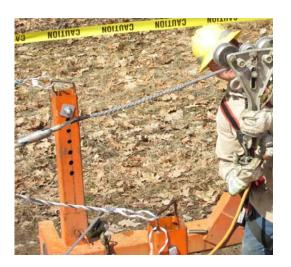
Next, the Kellem on the wire should be attached to the Kellem on the Bull rope using the appropriate size swivel. The Swivel is very important, as when the wire and rope are under tension, they will spin at different rates.
