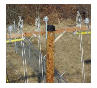
As with any work around hot wire, contact between energized conductors and hand lines, p-lines or bull rope is not allowed. For instances where incidental contact may occur, a barrier needs to be in place. The use of rubber cover up and/or the use of rubber gloves for a worker on the ground must be used.
