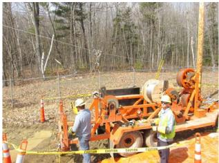
All grounds should be checked and running grounds, if used, should be installed. Once this is complete, the brakes should be released until the wire just starts to roll. The Rope Trailer can then be contacted and they can start to pay in slowly and start pulling the wire.
