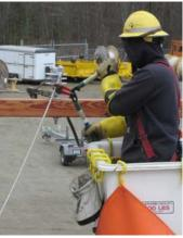
You want to make sure the wire end that is staying up is securely held with a hoist, hand line or other means before cutting down the conductor. Also, the workers on the next pole know you are cutting the wire down to them.
