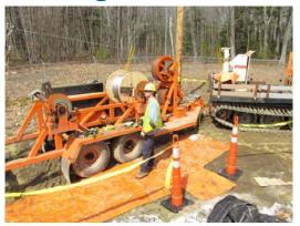
At this time, the brakes on the Wire Trailer can be adjusted as the wire slowly moves towards the first block.
