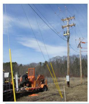
Positioning of both types of trailers is very important. Distance from the pole is an important consideration. It is recommended that the trailer be set back from the first pole a distance equal to 3 times the height of the pole.
