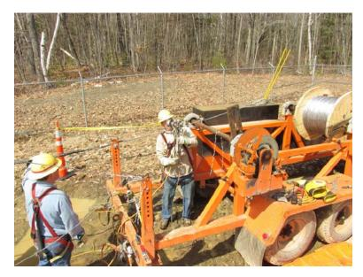
Also, a running ground and/or arbor ground needs to be installed to ground the conductor.
