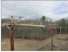
Another good practice is to tie in each phase as you move it to the hot arm. This helps to keep wire in place if a tree came down during the duration of the job and helps keep things in place in the future step of wire removal.
