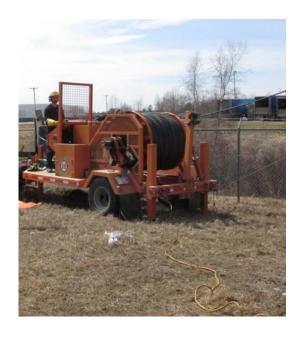
Then, the P-Line needs to attached to the Bull Rope with a swivel. The P-line will then need to be payed in and the Bull rope payed out either hydraulically or with the brake.
