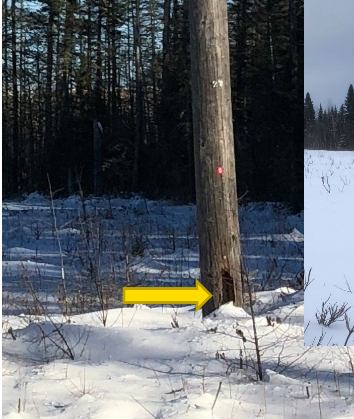
Rotted pole base, bear damage and leaning structure
